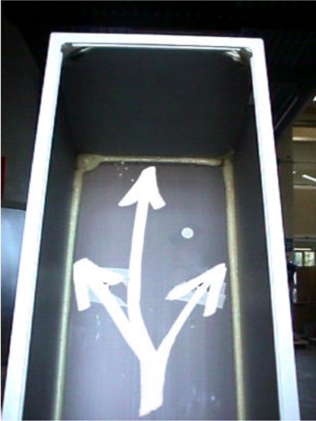
Picture 5: The flexible Polyurethane seal applied to the linear segments of the sealing pattern
