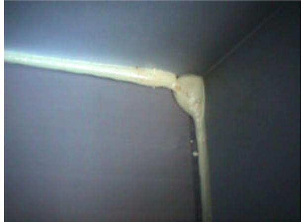
Picture 6: The flexible seal applied to the inner corners of the cabinet
